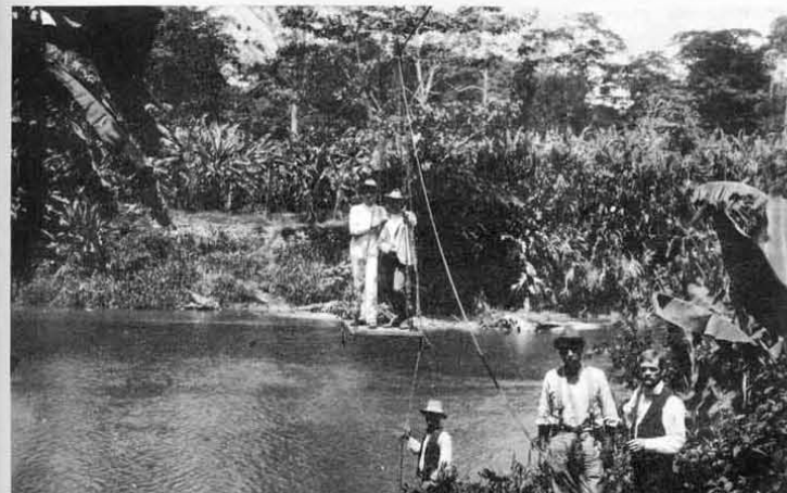
Cable-way for banana transport across Banana river (Beverly).
