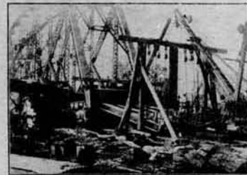
FIG. 2. LEVER RIG RAISING THE END OF REVENTAZON RIVER BRIDGE
