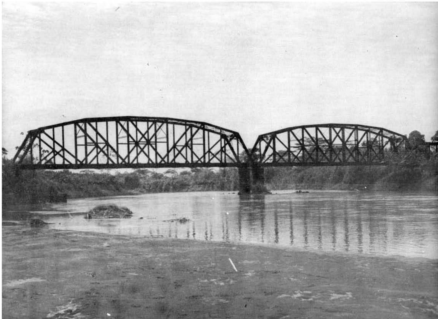
Longest bridge is the Matina river crossing. This photo shows two center spans and, dimly, one of the approach spans. Crossing consists of four through trusses and nine deck girder spans. Total length 1321 feet.
